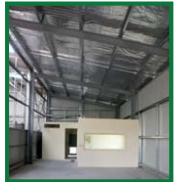
Refinery shed extension.
